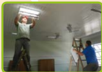
Upgrading of lighting systems at Roberto Schutz Elementary School
